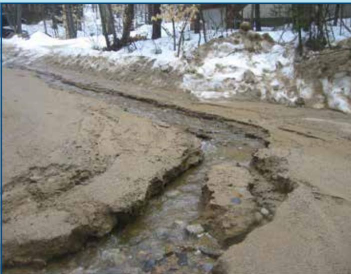
*Photo 1: Runoff water caused this rural road to be eroded away.*
